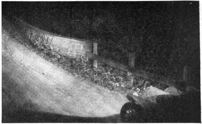
A stone wall and hill. The car is equipped with Rushmore Headlights, Searchlight and Generator.
